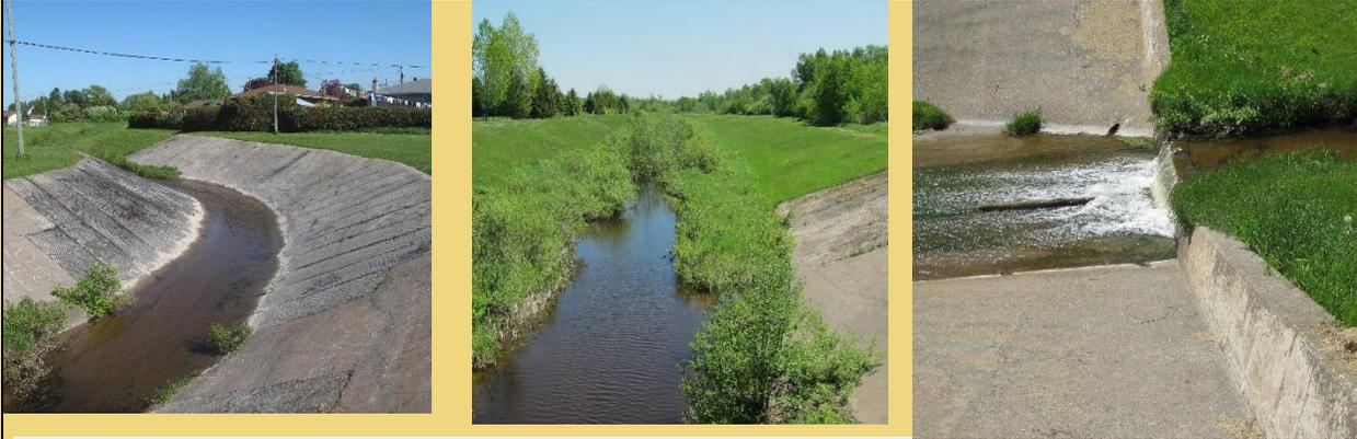
**Photos SSM – downstream - “grey infrastructure” to prevent flooding.**
