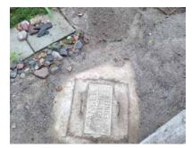
Property owners without access to municipal sewers must install and maintain their own sewage treatment system. Septic systems are most common. In these setups, anything that goes down the drain or toilet flows into a two-chambered underground storage tank that separates out solids. From there, wastewater is routed to a soil leaching bed that filters most contaminants. Proper installation, repairing, upgrading or replacing a rural septic system is subject to the Ontario Building Code.
