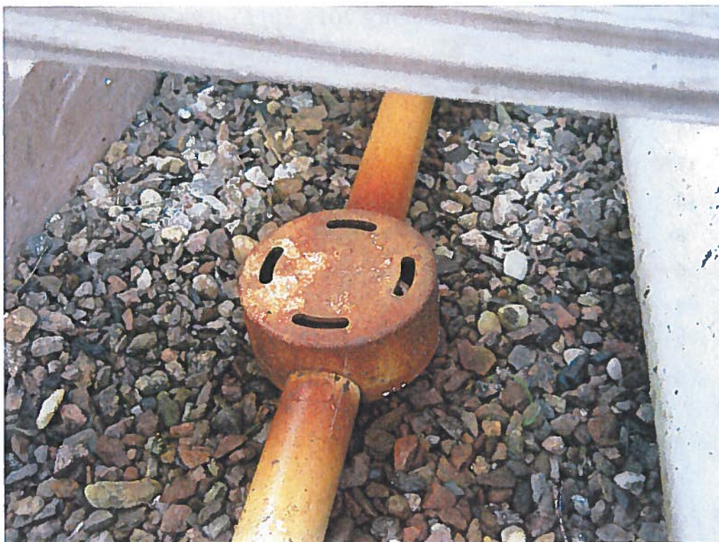
Figure 4. Iron oxide scale coating on distribution pipes and on upper pea gravel in the ETI recirculating sand filter.
